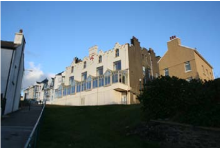
Photo 1: Change in level between the Promenade and Shore Road
