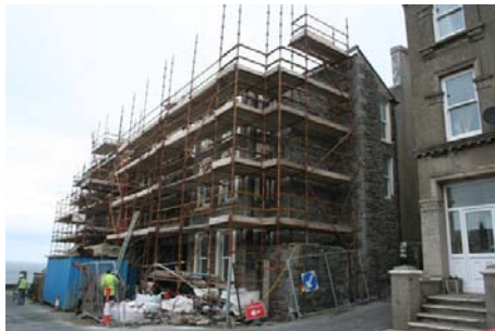
Photo 29: New building replacing Bay View Hotel
