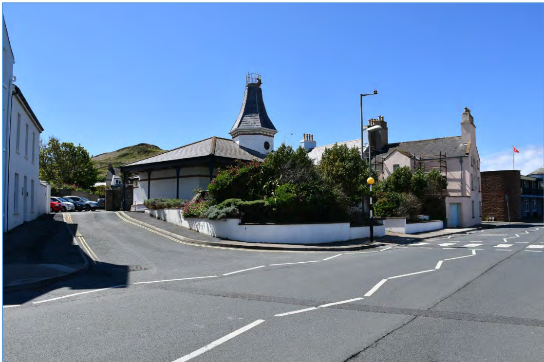
Photograph 23 – Peel Sewage Pumping Station Works, Shore Promenade, Peel
