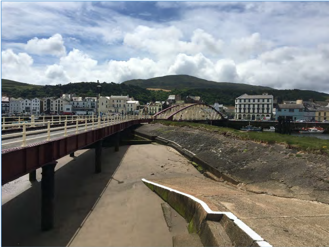
Photograph 1 – showing the Swing Bridge and harbour, with quayside buildings
