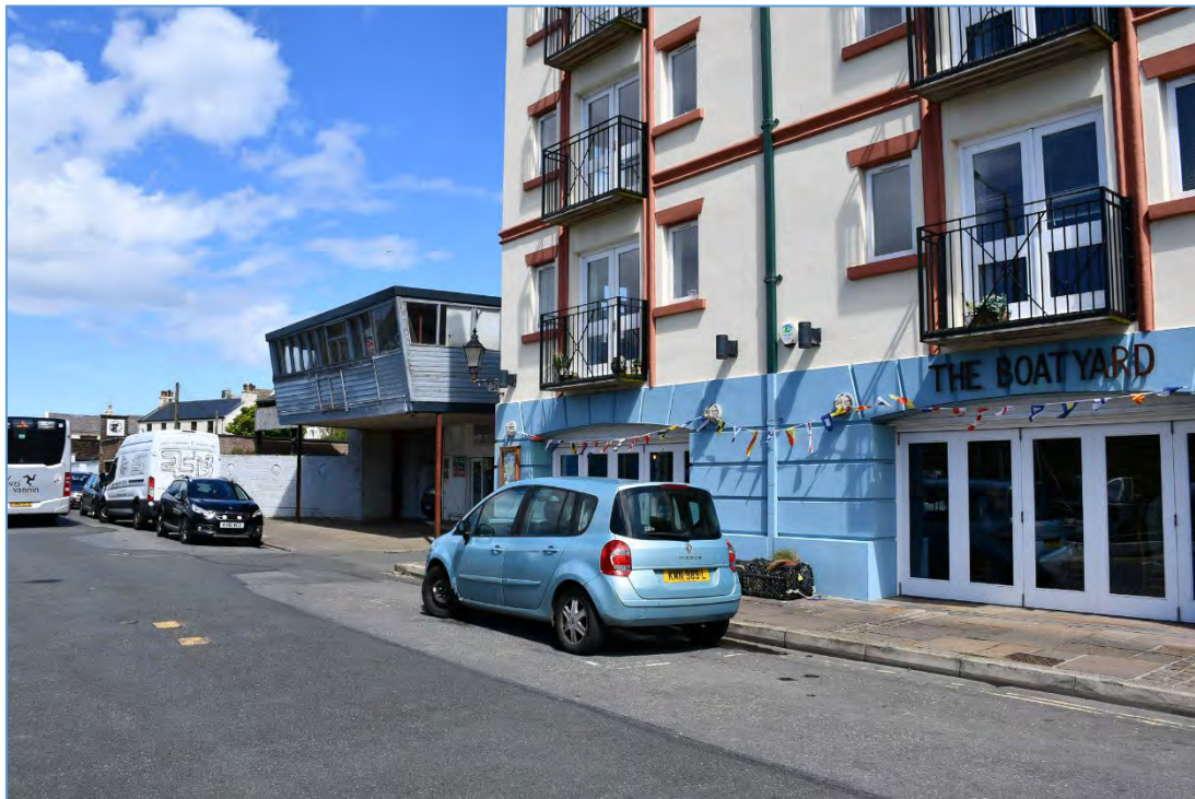
Photograph 16 – The Boatyard adjacent to the former garage (now vacant)
