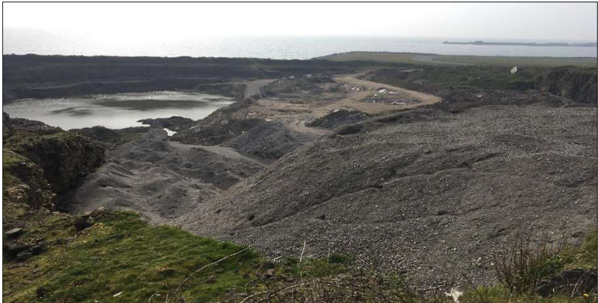
Plate 3. View of NTL from north-west edge of quarry (April 2019)
