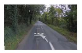
The A5 is an important primary route linking the south of the island to Douglas. The section between Santon Motel and Fairy Bridge has poor geometry, visibility, running surface and drainage. Tests on the existing carriageway indicate that both the surface and foundation are failing and require complete reconstruction.
