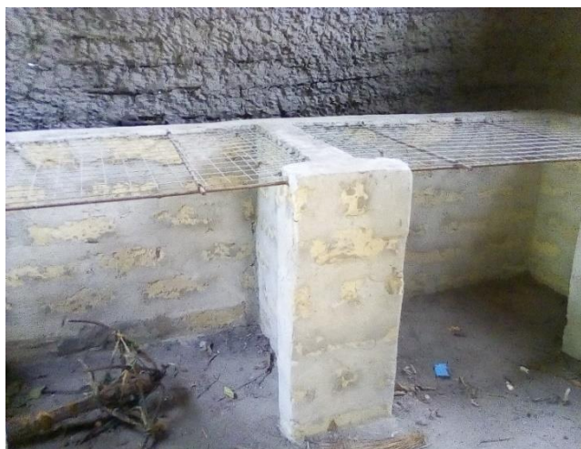
Internal and External views of one of the fish smoking Chorkor Oven constructed by the project.
