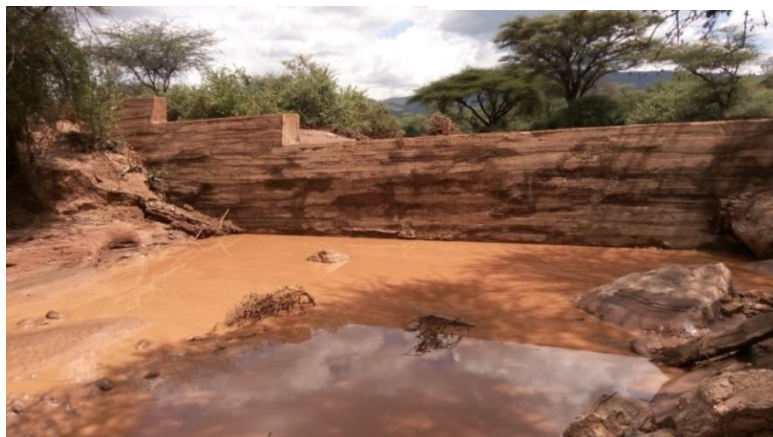
Completed New Picnic Dam funded by the Isle of Man IDC 2014 Small Grant
