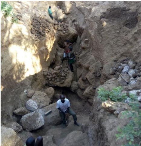
Excavating bedrock ahead of construction
