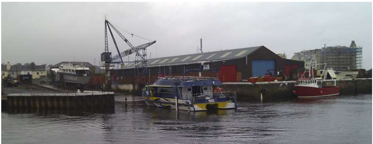
Ramsey Shipyard. Photo: Department of Infrastructure.
