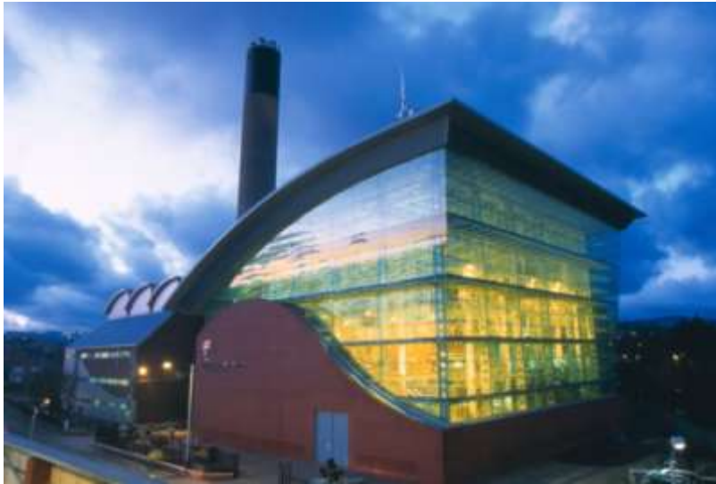
Pulrose Power Station, Douglas. Photo: Manx Utilities.
