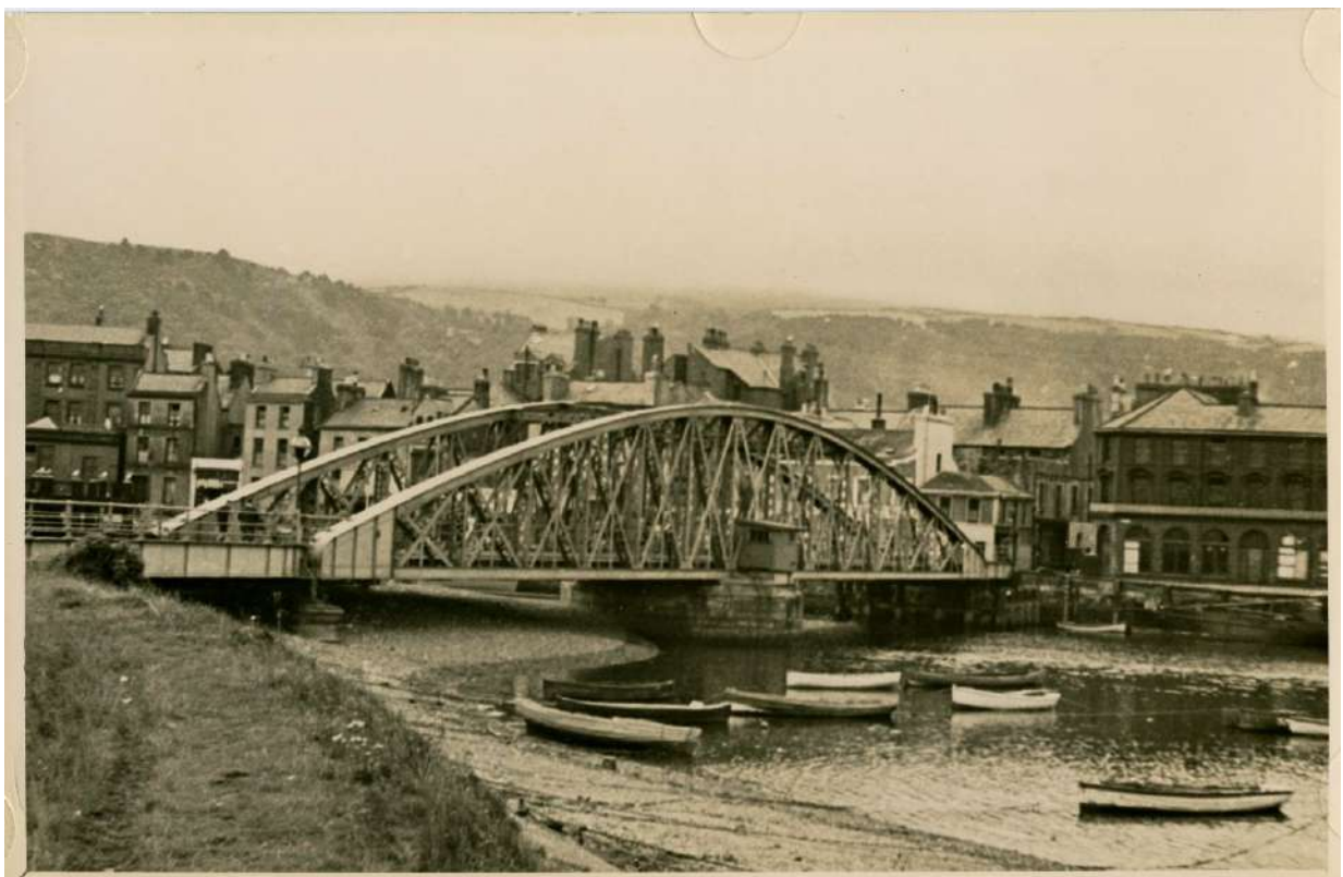
Image of Swing Bridge – dated 1948
