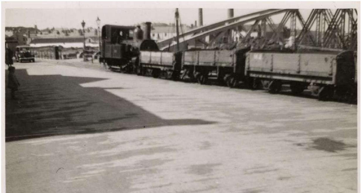
Image showing train on harbour branch with Swing Bridge behind – dated 1946
