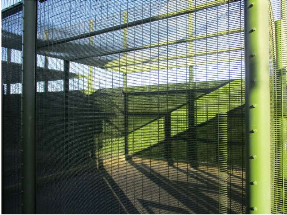
Segregation unit exercise yard
