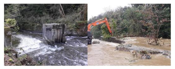
Photograph 7 - MER weir and sluice gate superstructure in the River Laxey, before removal. (Gap B), nearside of wall is Glen Road.
