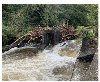
Photograph 2 - Accumulation of debris behind the MER weir on the 1 October 2019
