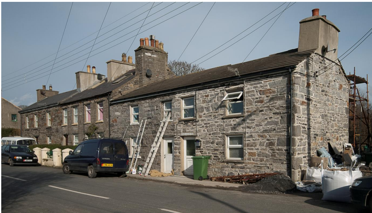
Limestone cottages north of the stream running through Ballabeg, some with traditional gateposts
