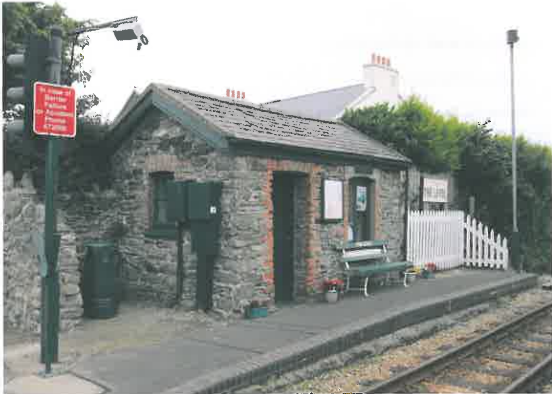
West and south elevations during August 2013. Note the additions since the previous 1966 photograph; low level platform, bench, barrier control cabinets, picket fence and station nameboard.
