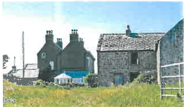
Scarlett House and farm. The step pitch of the double pile roof is clearly saeen in this view. 12.6.2008
