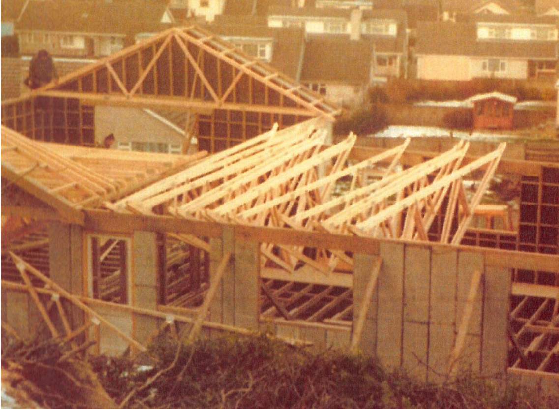
Property under construction
