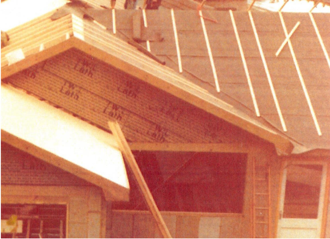
Property under construction
