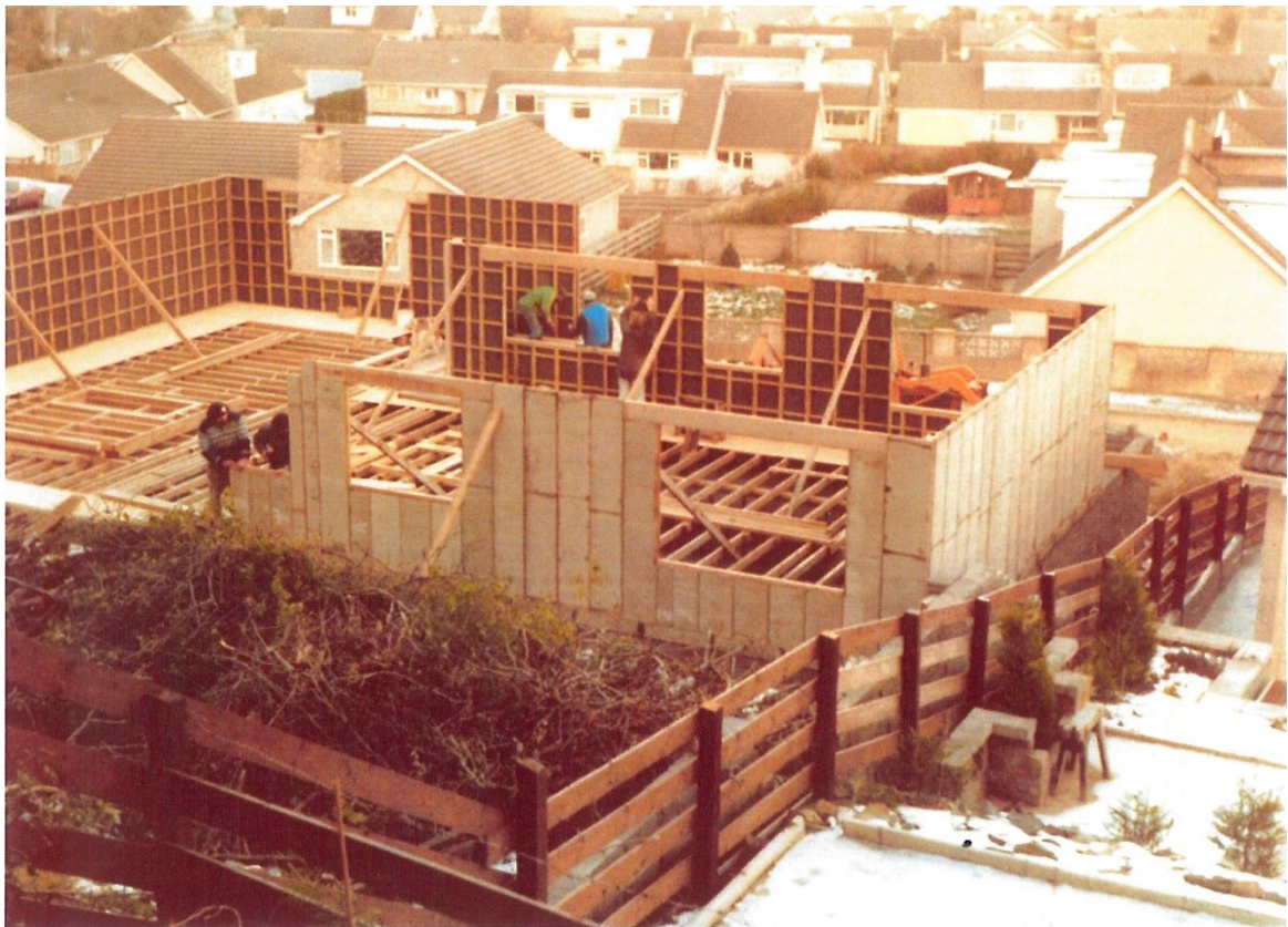
Construction of property
