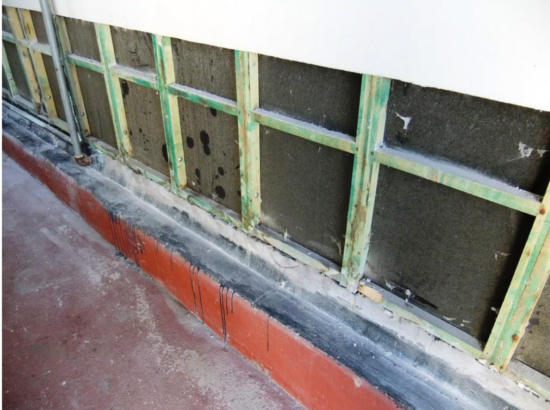
Garage external wall panels exposed during alterations in 2014
