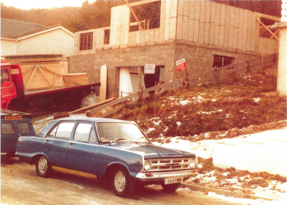
Construction of property
