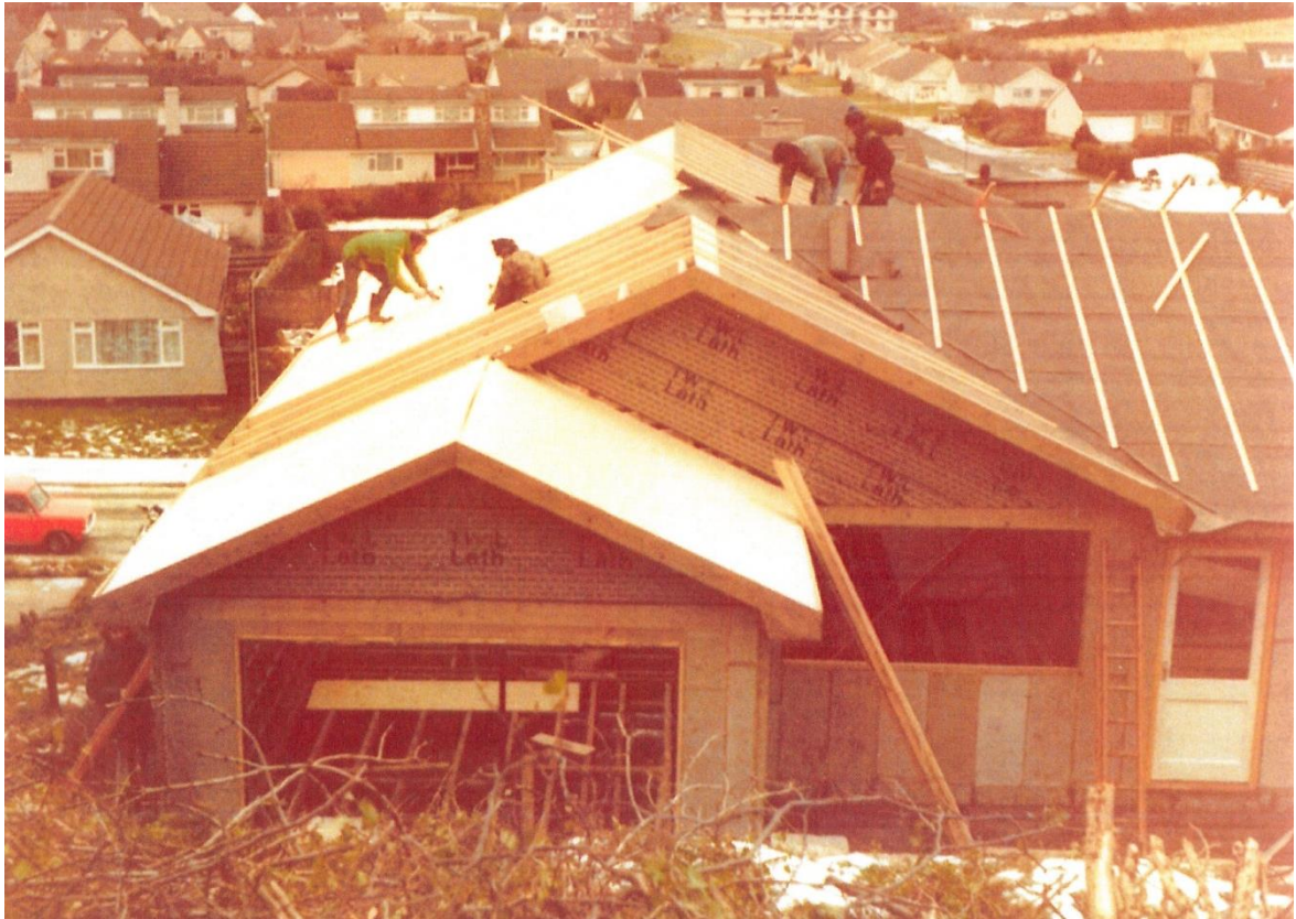
Property under construction
