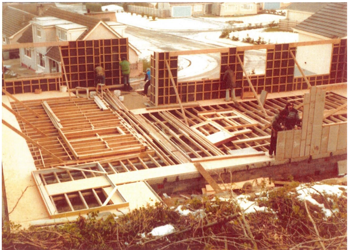
Construction of property
