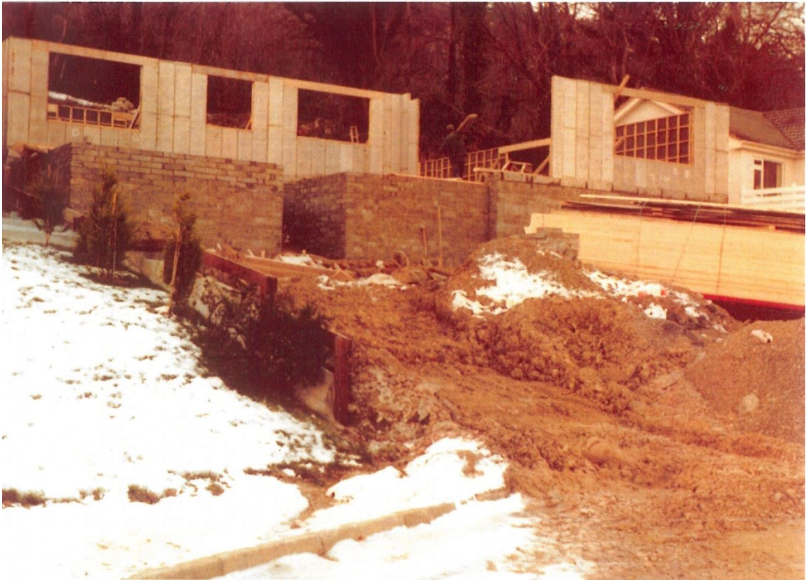
Construction of property
