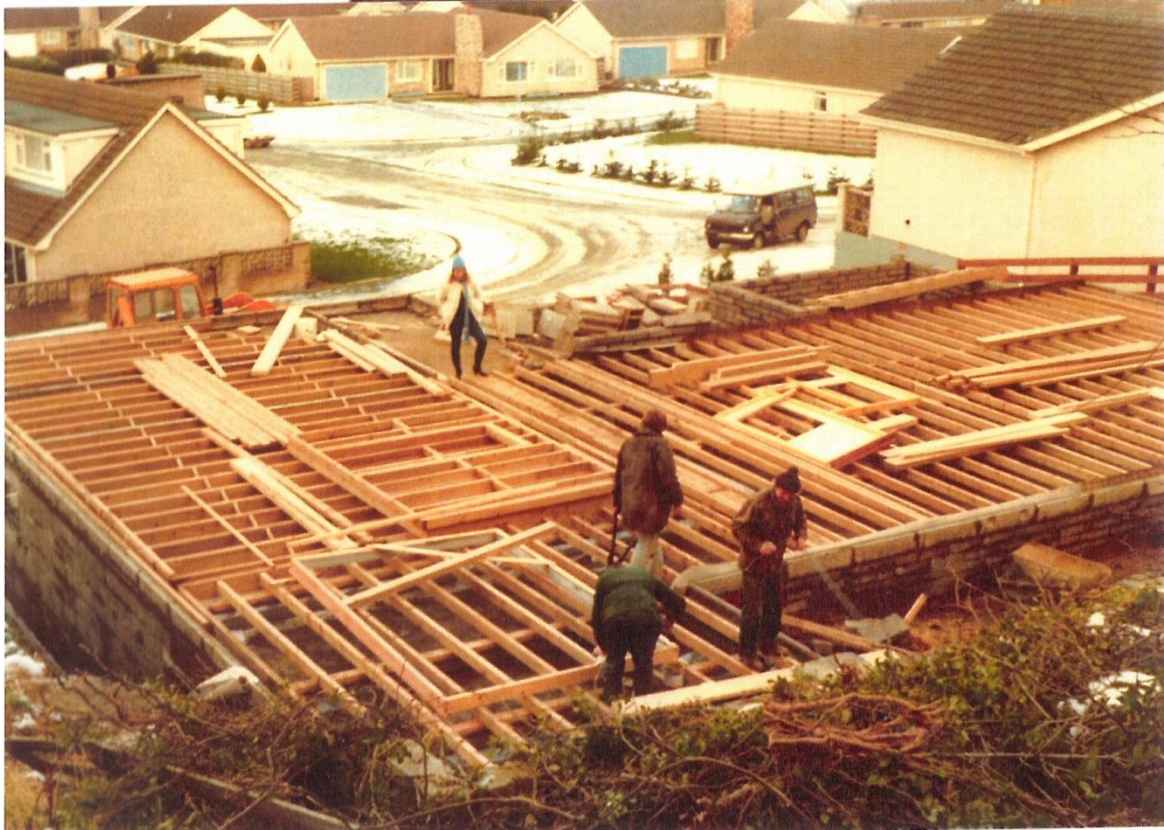
Construction of property
