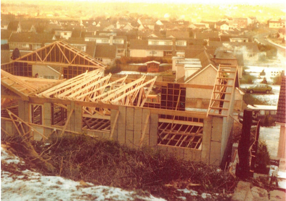
Construction of property
