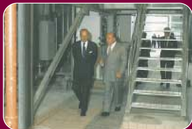
Chief Executive Mike Proffitt and HRH Duke of Edinburgh in the new Turbine Hall at the CCGT Pulrose Plant.
