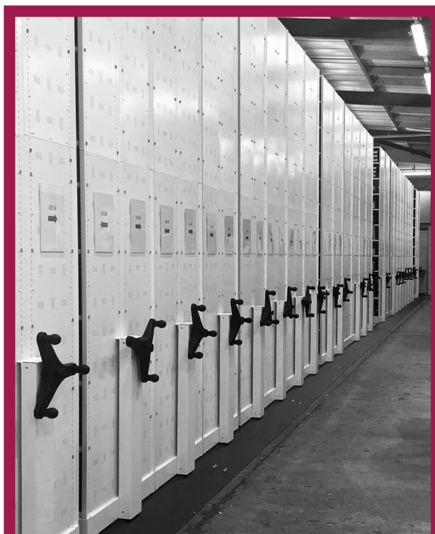
After: New mobile shelving (sufficient for storing 670 cubic metres of archives)
