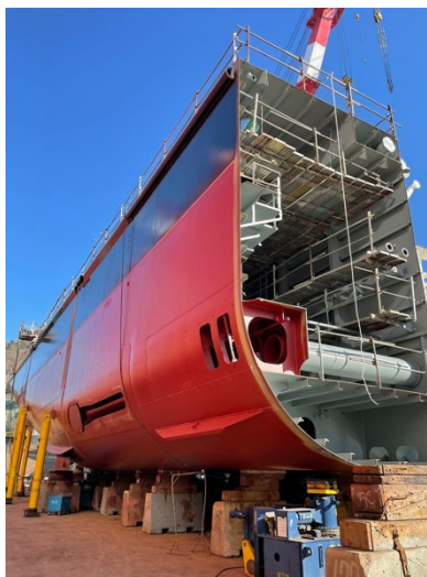
The Manxman construction
