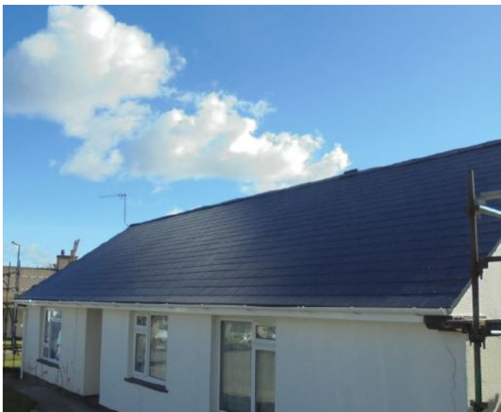
Refurbished properties at Ayre View
