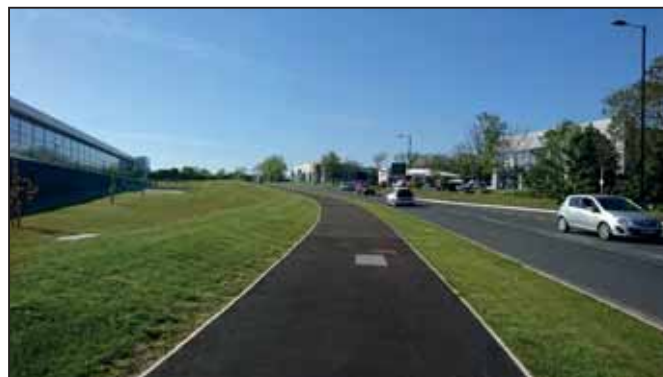
11. Isle of Man Business Park developing infrastructure
