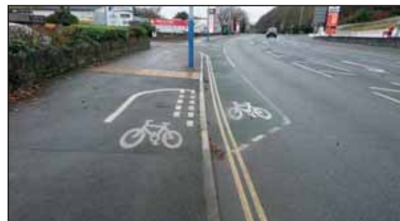
Figure 7. Peel Road cycle lane
