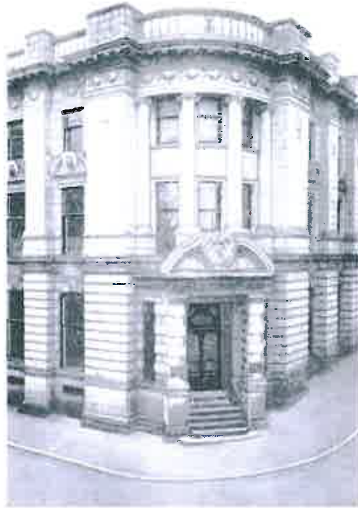
Head Office, Atholl Street
