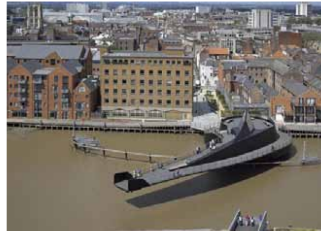
Hull swing bridge is both functional and an attraction, allowing passengers to ride it whilst it is motion.
