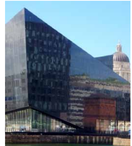
Mann Island, Liverpool – A landmark waterside development on the dockside.
