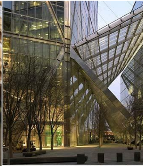
Broadgate, London - A covered street gives shelter to space and provides a recognisable feature.
