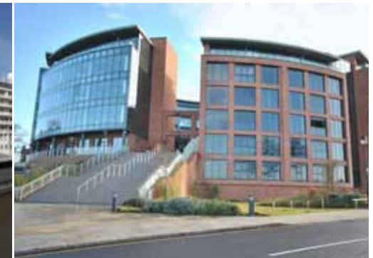
HQ building, Chester, creates an enclosed public space within the core of the buildings.
