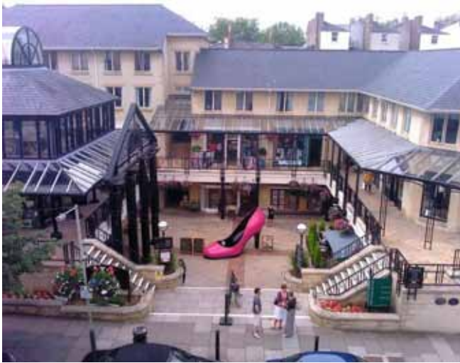
Cheltenham Montpellier Courtyard – the creation of active space and a cluster of boutique retail.
