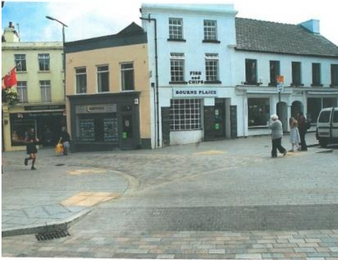
Ramsey – shared space scheme using high quality materials highlights the positive effect of public realm investment on placemaking.
