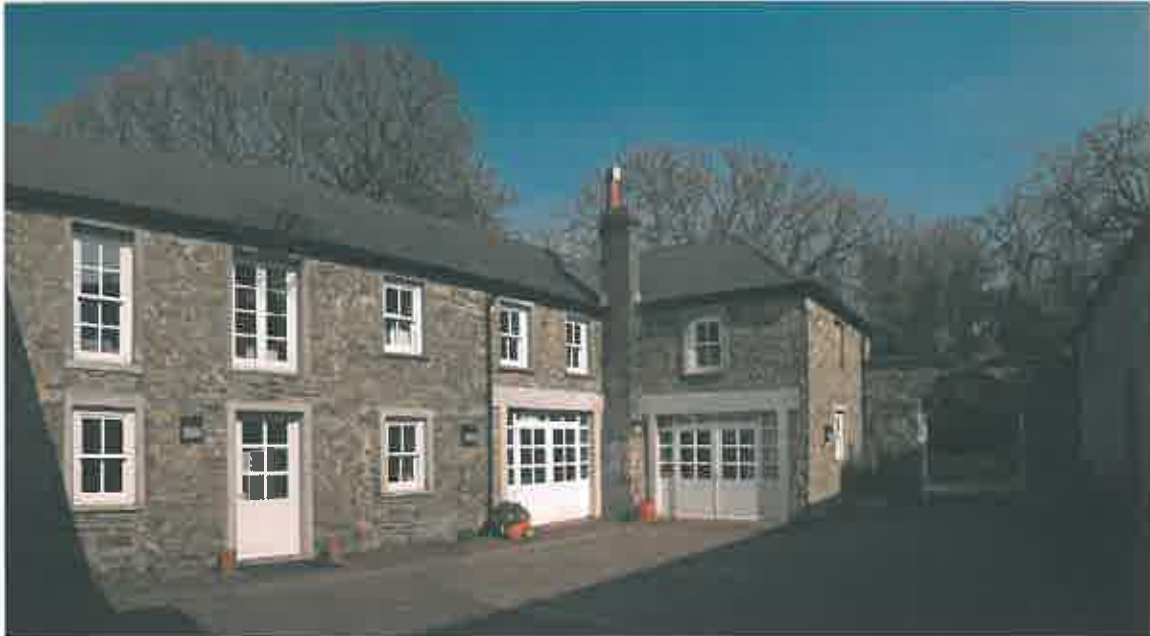
Stable Building PAT/19.3.2015
