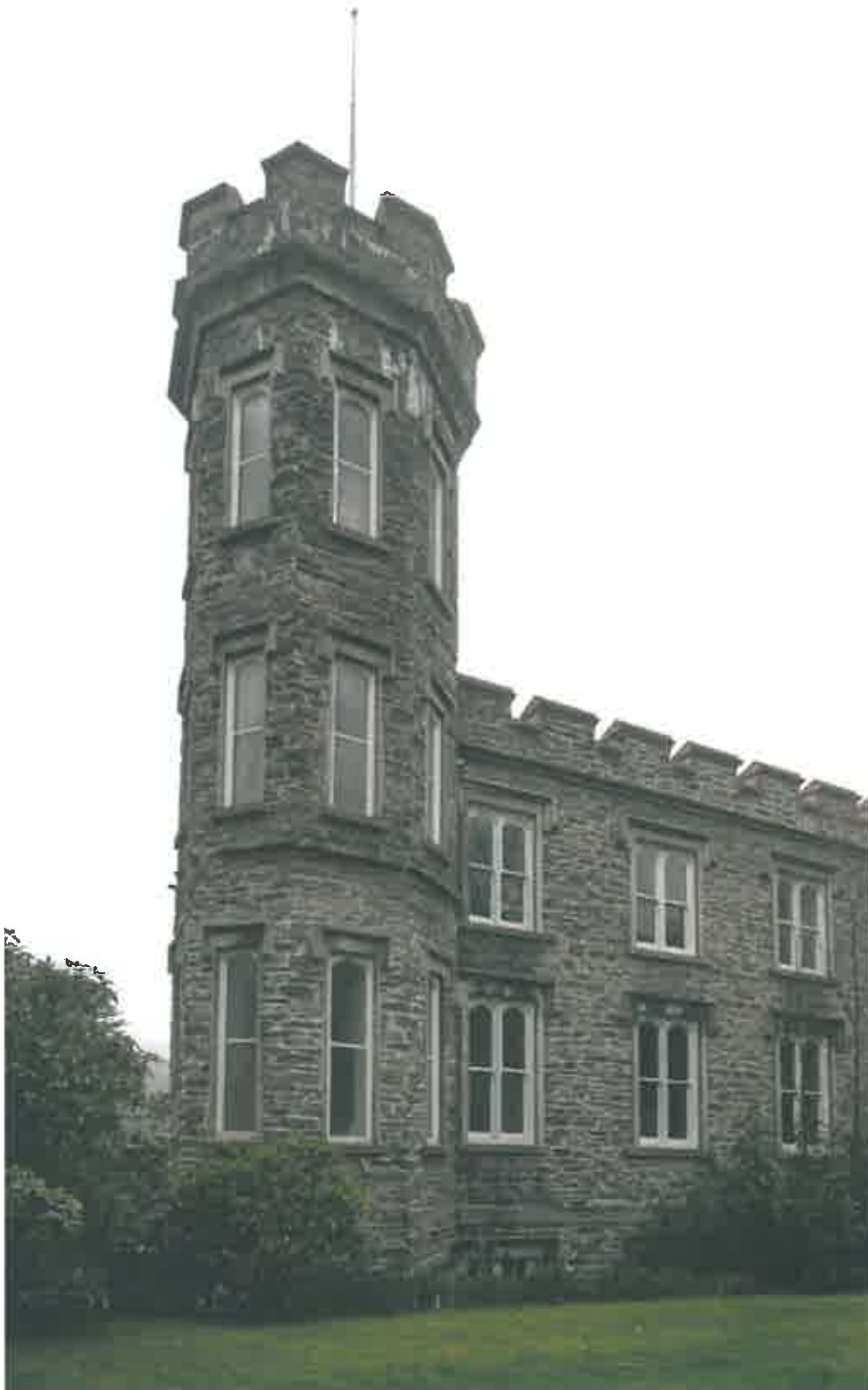
Above left: the Tower – a larger version of the false chimneys, with windows. The hood mouldings do not have a return stop. Note the slate damp proof course below the first floor windows. PAT/6.4.2015
