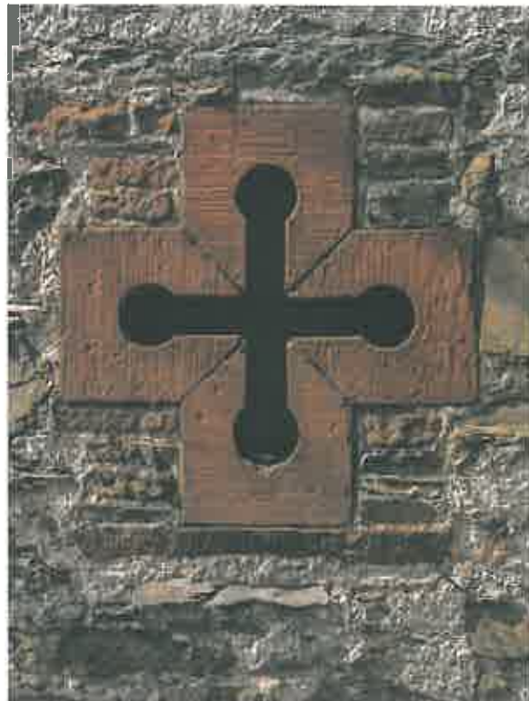
One of the four false arrow-loops symmetrically disposed about the entrance door and the window above it, in the east elevation of the Stable Building. PAT/9.4.2015
