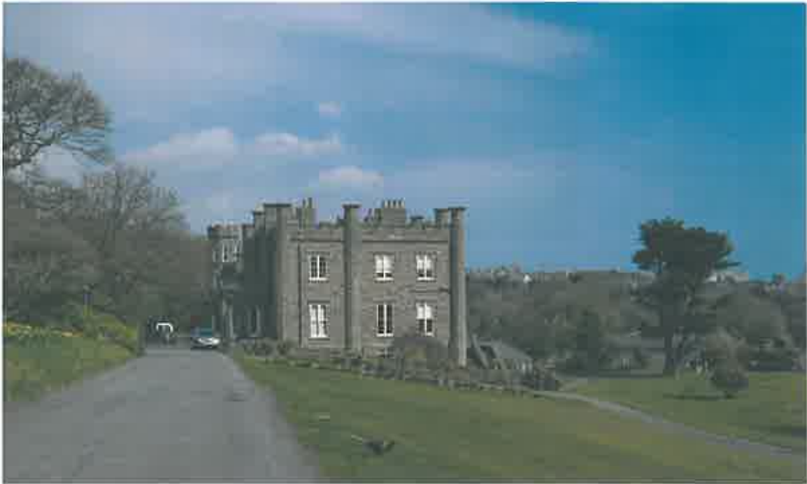
View of the west elevation from the carriage drive. Pat/
