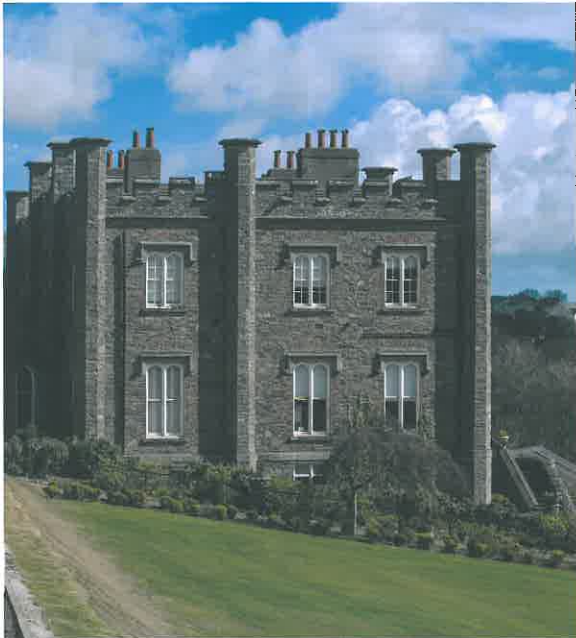
The east elevation, clearly showing how the building has been set into the slope of the ground. PAT/12.4.2015
