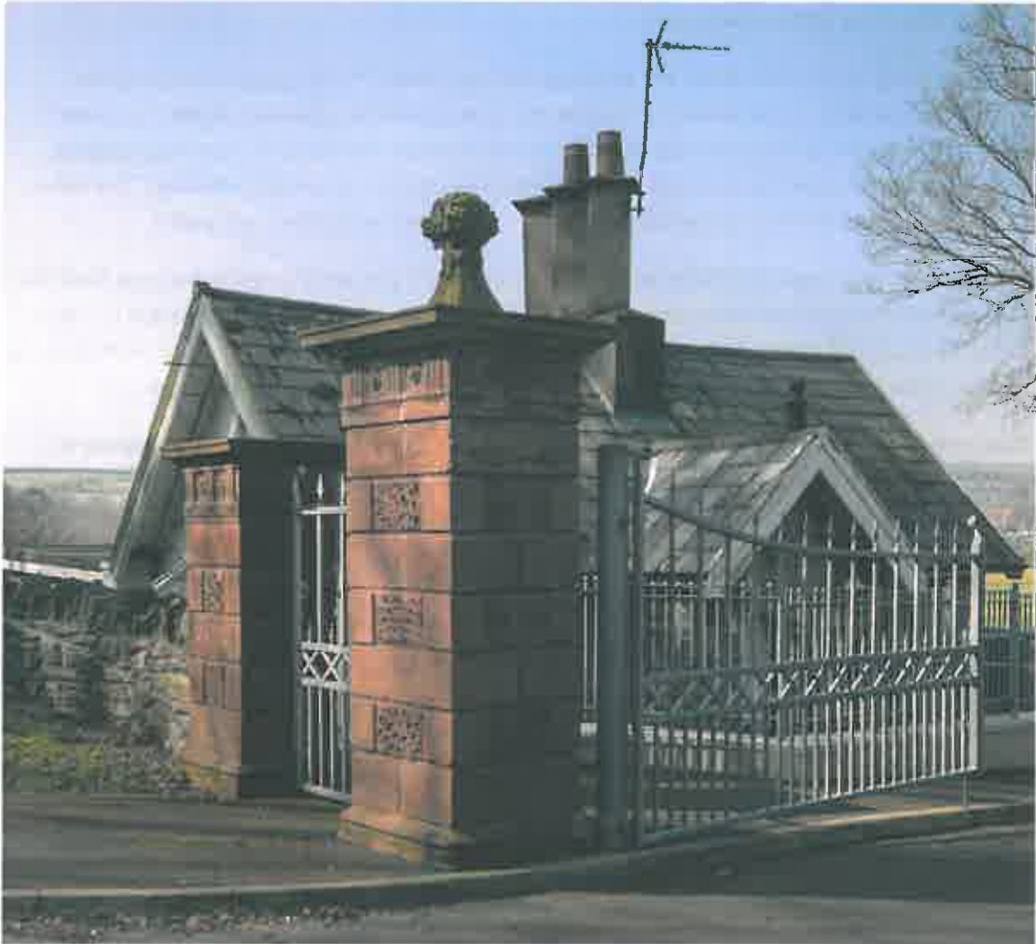
The gateposts were badly damaged in a road traffic accident in 2010 and carefully restored. In red sandstone with a Greek frieze under the capping and rustication to some of the stone work. The two larger gateposts are surmounted by carvings representing elements of the Taubman crest. PAT/
