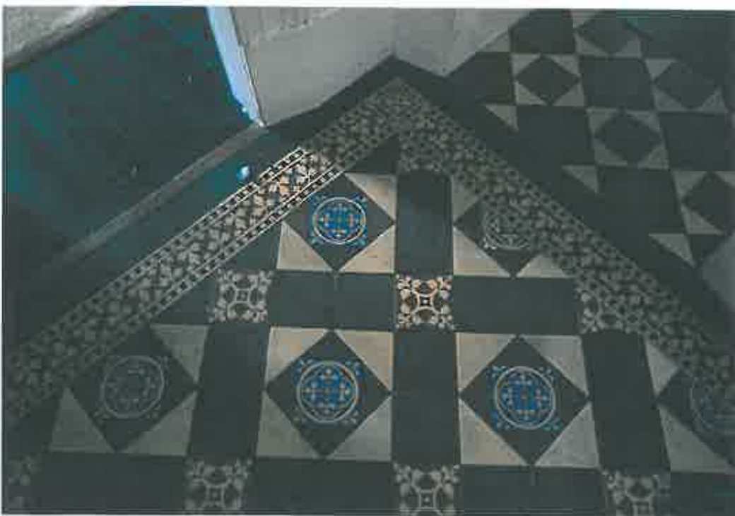
All the tile designs used in the hall can be seen at the corners of the room, where it is evident that the proportions of the hall were not designed to suit the tile pattern. The door threshold on the right uses smaller plain tiles; the narrower threshold on the left is marked by a narrow strip of terracotta tiles.
