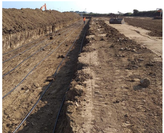
CRHS New Pitches – laying the ground source pipe arrays
