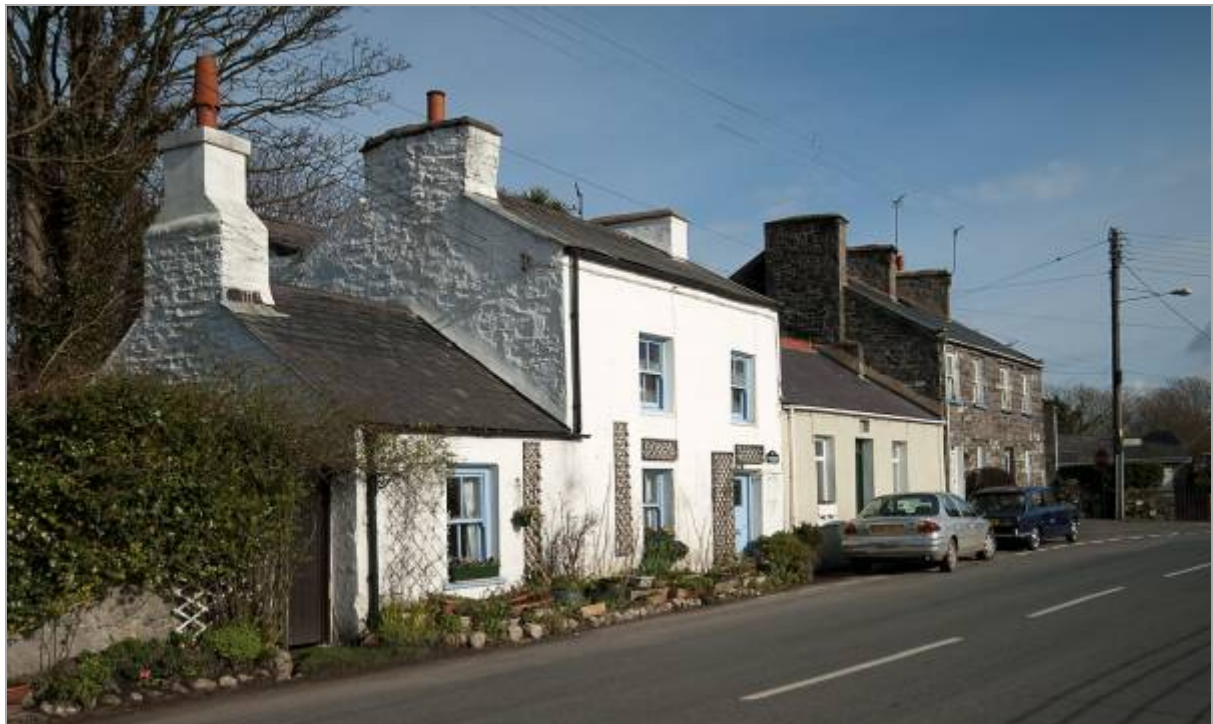
Cottages to the left of the view in the top photograph. A dynamic little group of one and two-storeys. Only the end cottage, adjoining the Grenaby Road junction, remains un-rendered limestone.
