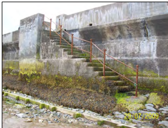
Photo 4 – Access steps to the beach
