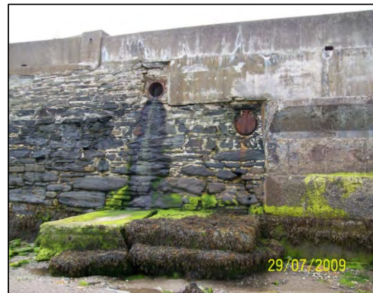
Photo 5 – Drains in sea wall
