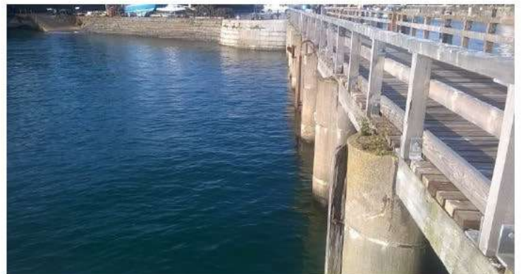
Figure 12: Area for disabled people's access pontoon
