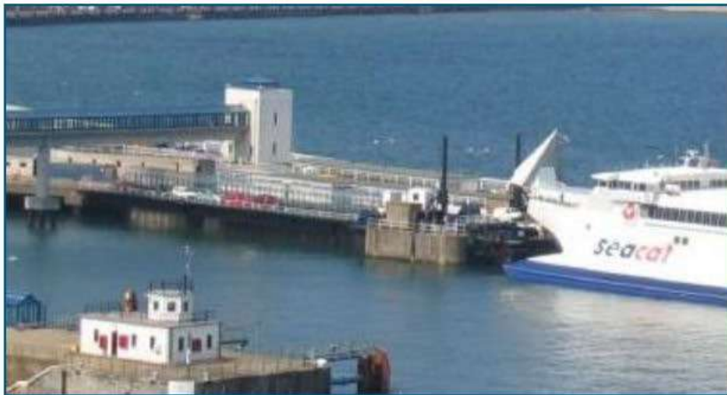
Figure 4: Existing vehicle linkspan to Queen Victoria Pier
