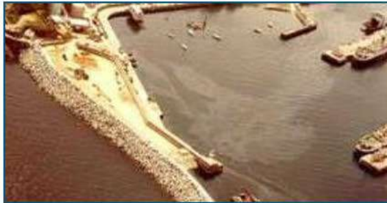
Figure 16: Aerial view of the tanker Berth
