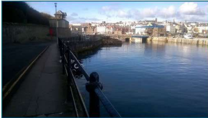
Figure 9: View of the Middle Harbour towards the Bascule Bridge
