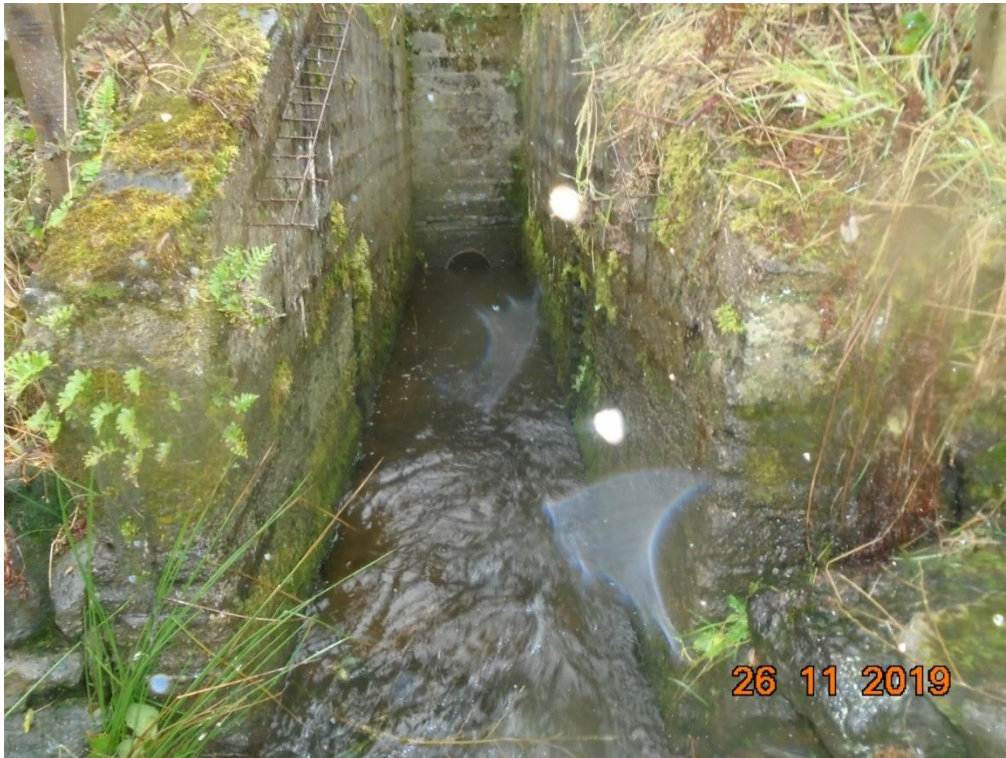
Photograph 9: Upstream headwall and overflow/outlet structure.
