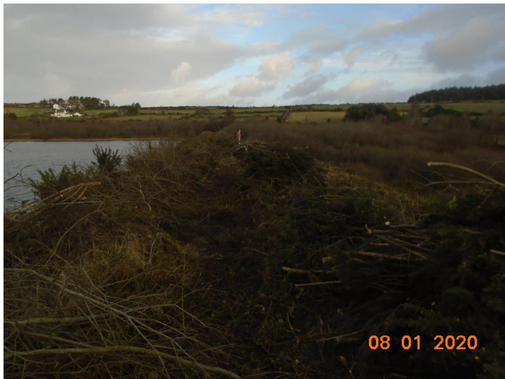
Photograph 7: Crest of eastern embankment.
