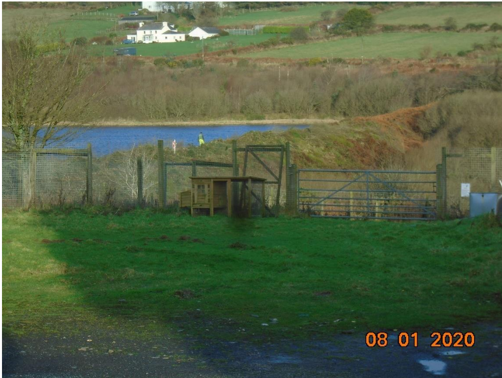
Photograph 5: Upstream face of eastern embankment.
