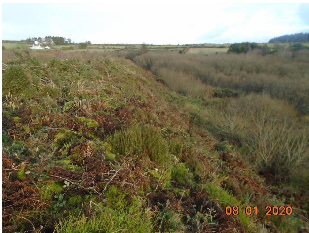
Photograph 8: Downstream face of eastern embankment.
