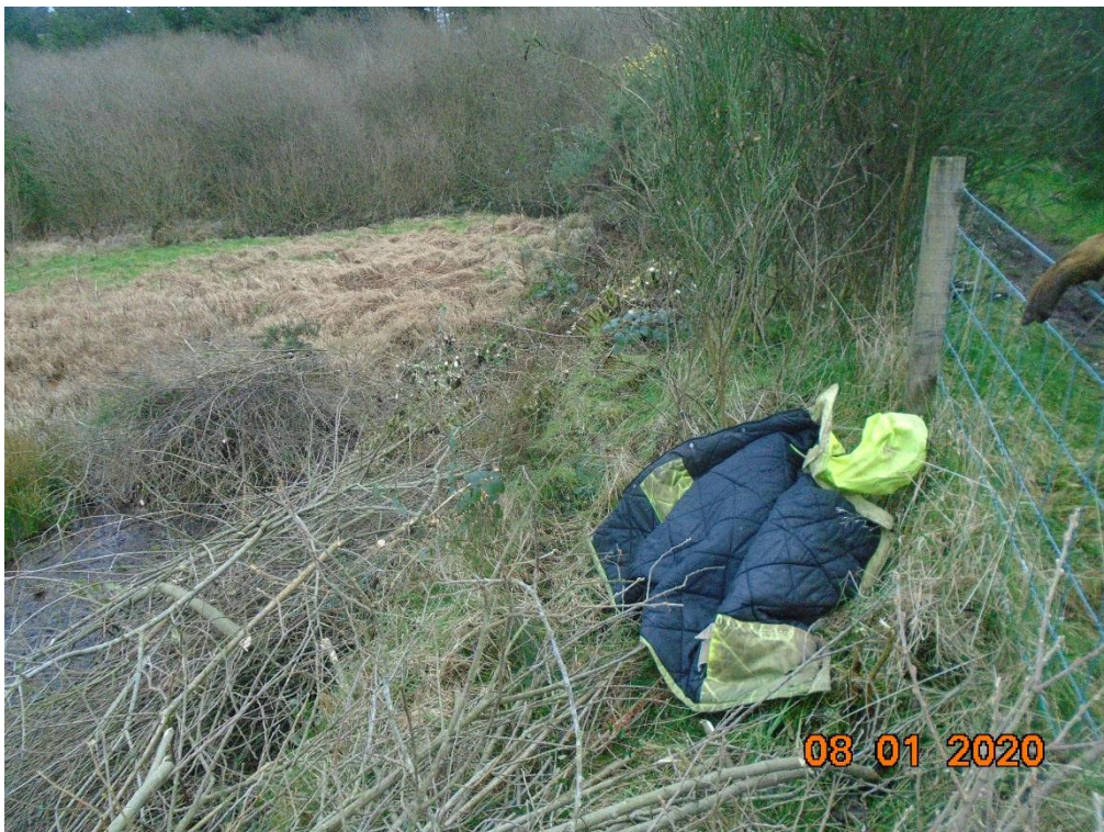
Photograph 2: Upstream face of the western embankment.
