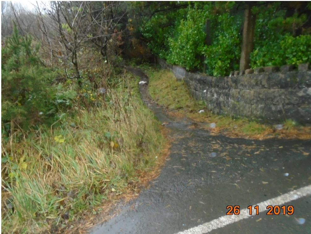
Photograph 11: Footpath/cycleway access to western embankment from A24 Foxdale Road.
