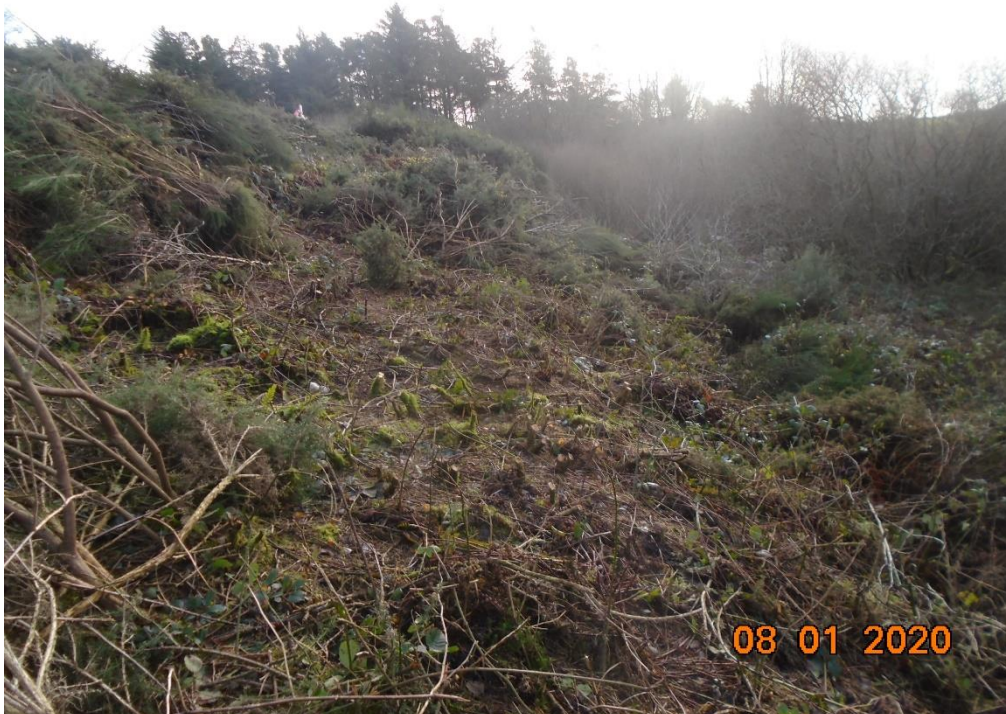
Photograph 4: Downstream face of western embankment.
