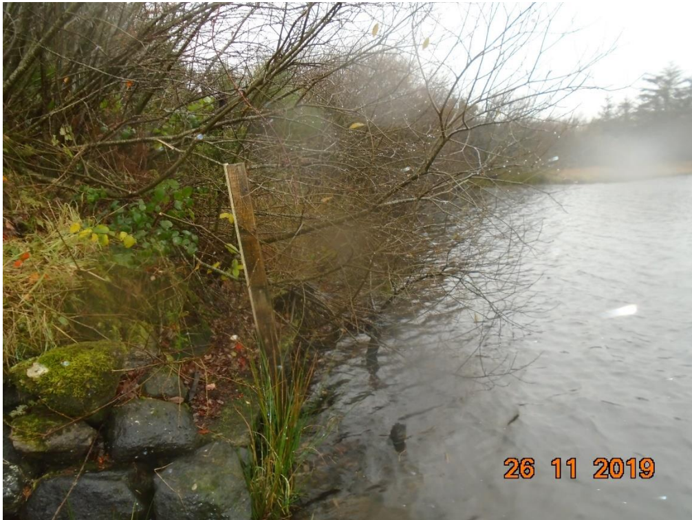
Photograph 1: Upstream face of the western embankment.
