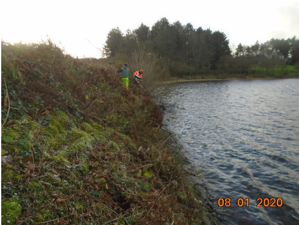
Photograph 6: Upstream face of eastern embankment.
