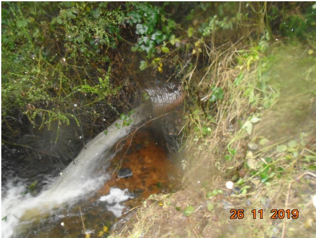
Photograph 10: View of downstream overflow outlet.
