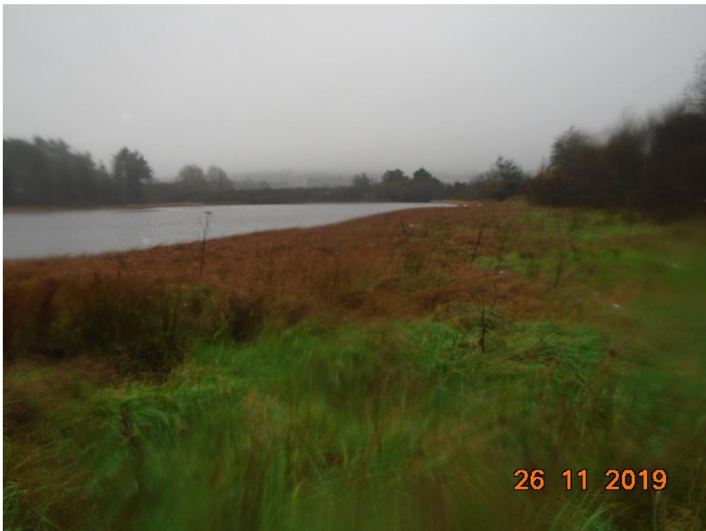
Photograph 14: Bankside area – north-western side of reservoir.
