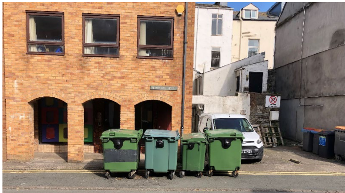
Fig. 16: Photograph to show Market Street rear elevations
