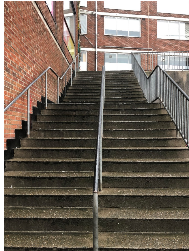
Fig. 11: Photograph to show steeped access
