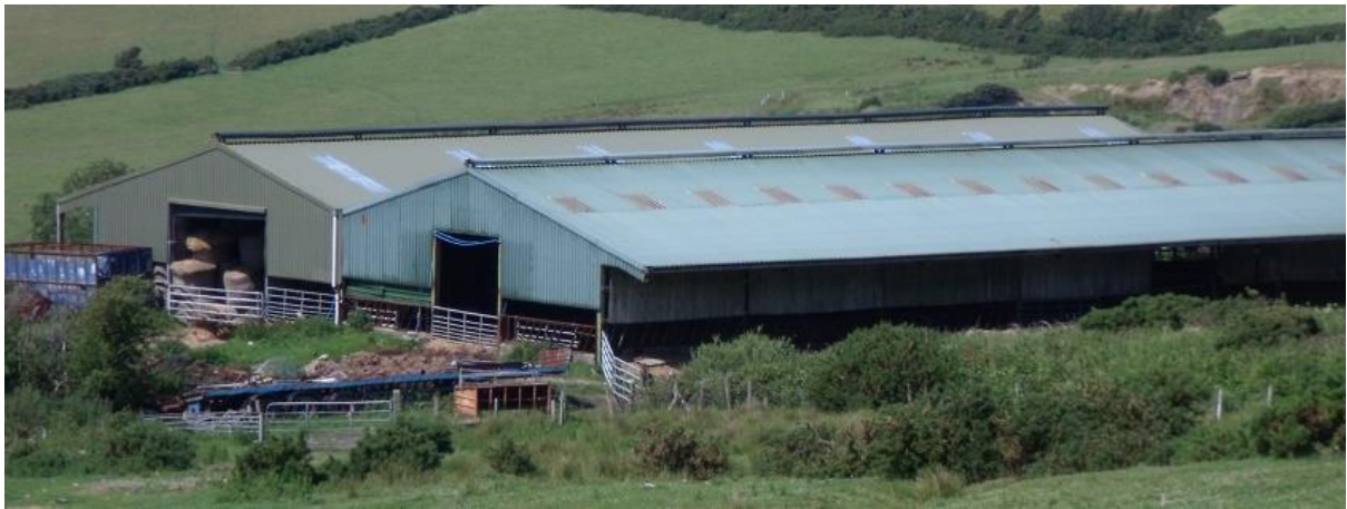
Figure 4: This shows a multi-span building each of which has its own protected open ventilated ridge.
