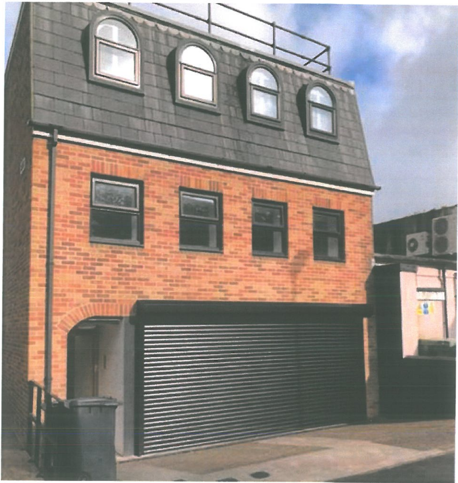
Rear of Property fitted with insulated garage door
