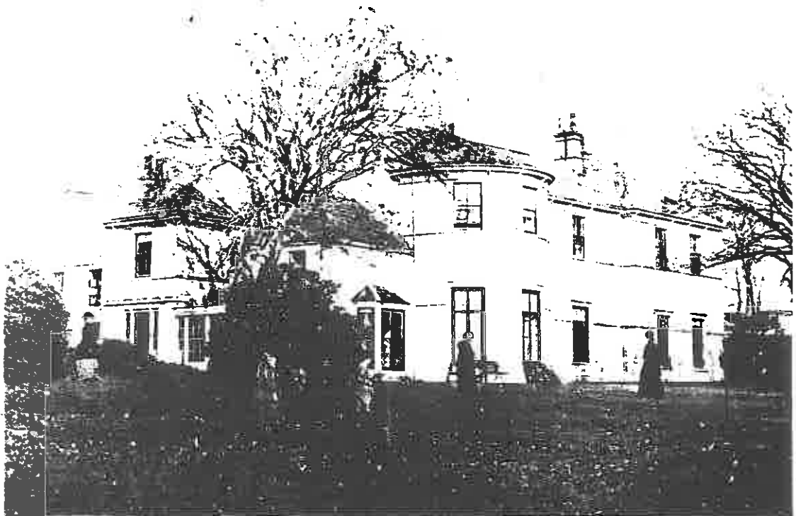
Bemahague, about 1885, showing alterations and extensions. (James Fenton)
