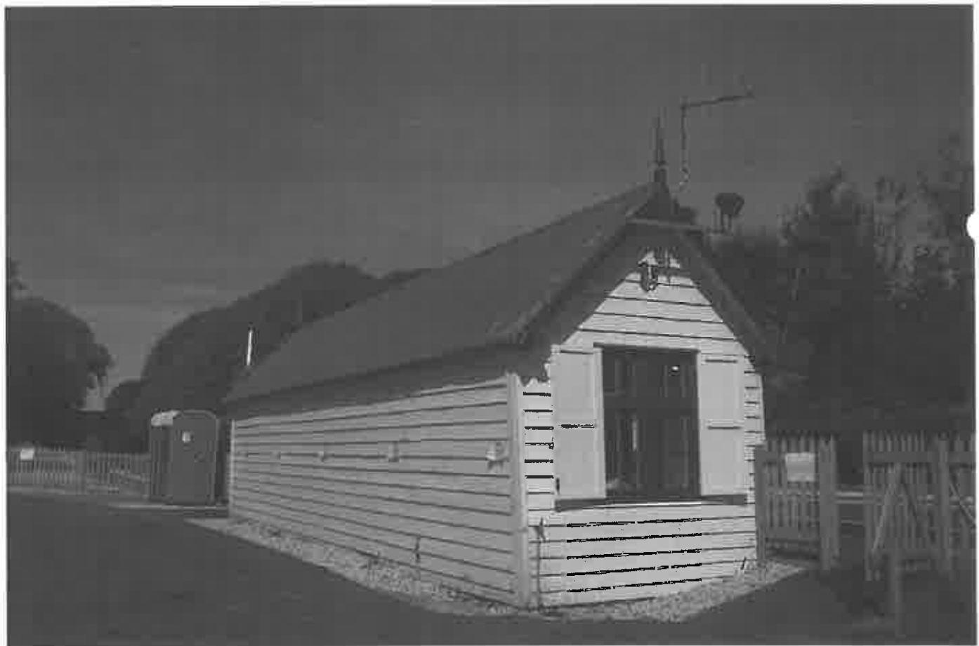
The rear of Santon Station Building looking north east.
