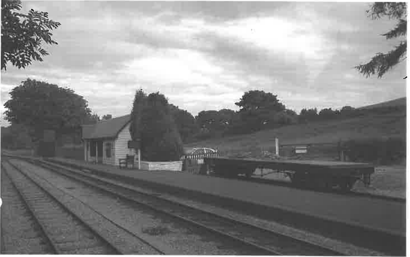
Two general views to capture the ambience of the station site; this photograph is from the Douglas bound platform looking South West.
