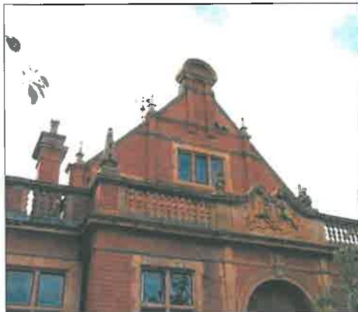
Peel Police Station front gable
