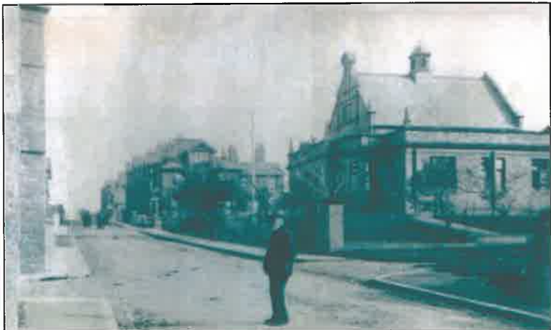
An early photograph showing the Court House complete with railings. (Leece Museum, undated)
