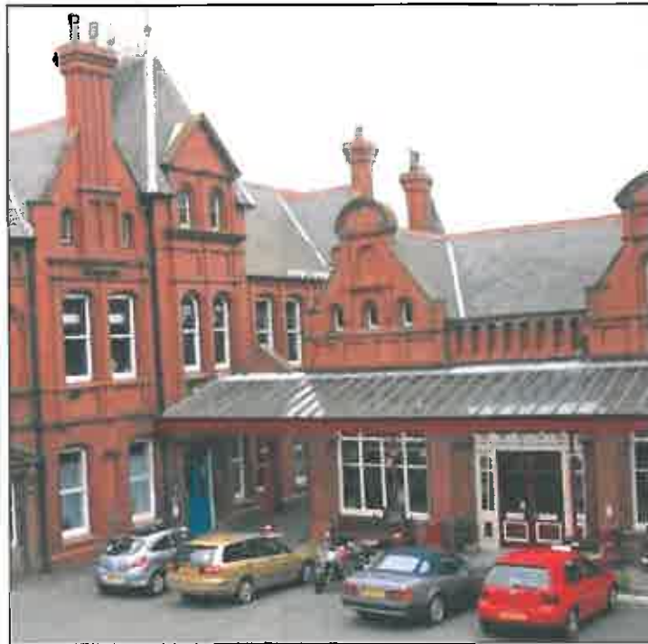
Pilasters and rounded gable details. Douglas Railway Station
