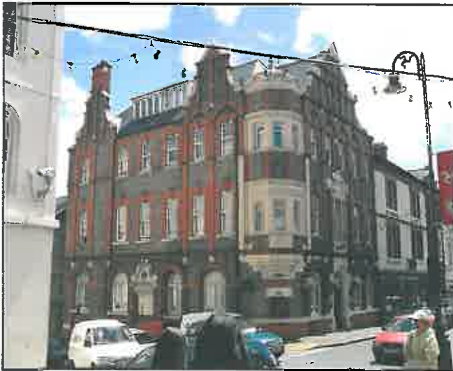
Former Ridgeway Public House, Douglas notable for its Dutch inspired gables and terracotta panel of sunflowers - a highly stylised image associated with both the Arts & Crafts Movement and the Aesthetic Movement
