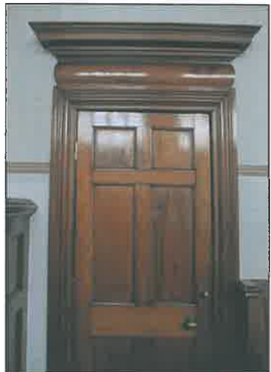
One of the fine examples of doors and frames which all have the same treatment, with a pulvinated moulding between doorcase and entablature.
