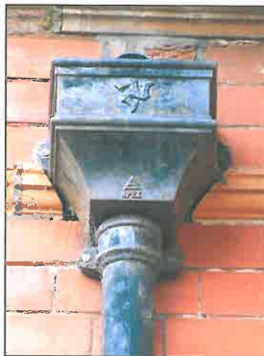
Rainwater hopper with distinctive three legs motif
