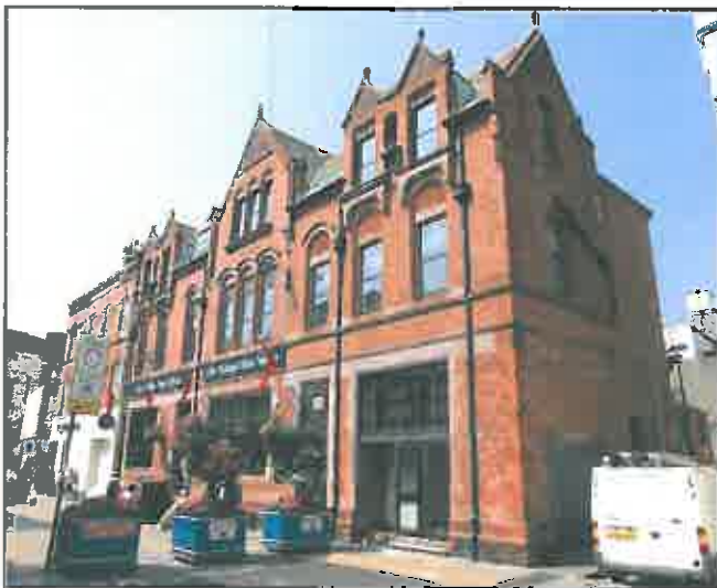
Douglas main Post Office, in addition to its use of Ruabon brick it is notable for its numerous moulded terracotta panels
