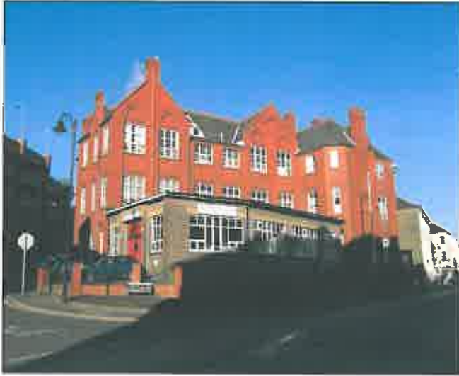
Former Hanover Street School, Douglas. Terracotta cast detailing forms the main panel by the front entrance
