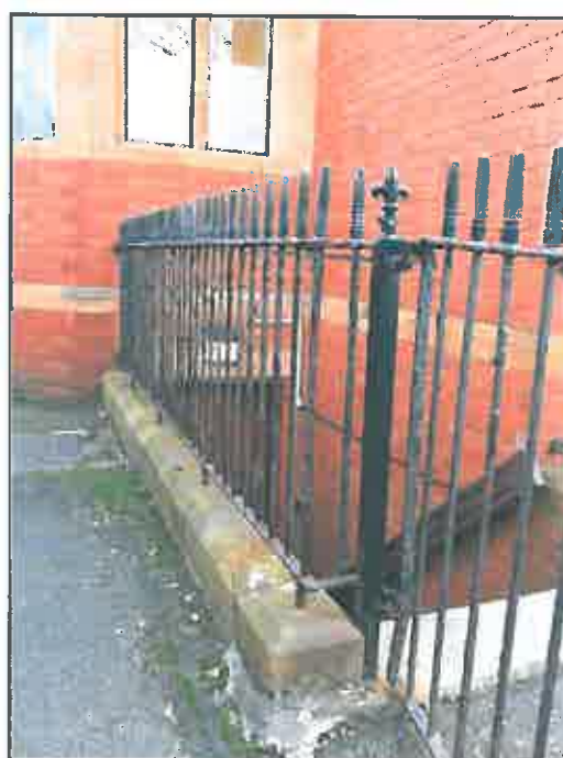
Rear elevation basement and railings which exhibits the only remaining sections of railing. Note replacement top sections
